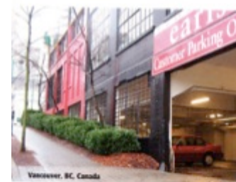
parking below the building
